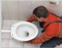
TOILET BEDDING AND OTHER PIPEWORKS
