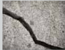
PATCH AND CRACK REPAIRS
