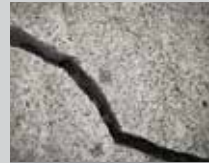
PATCH AND CRACK REPAIRS
