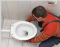
TOILET BEDDING AND OTHER PIPEWORKS
